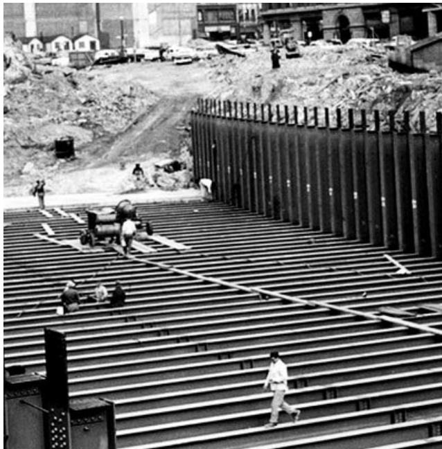
1956 Construction of Central Artery highway tunnel cutting through Chinatown, steel beam structure being laid, Boston Public Library.
