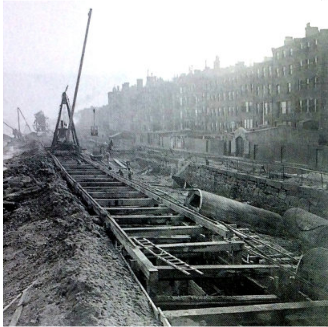
1908 Construction of seawall with sewer conduit, Back Bay, typical crane construction.
